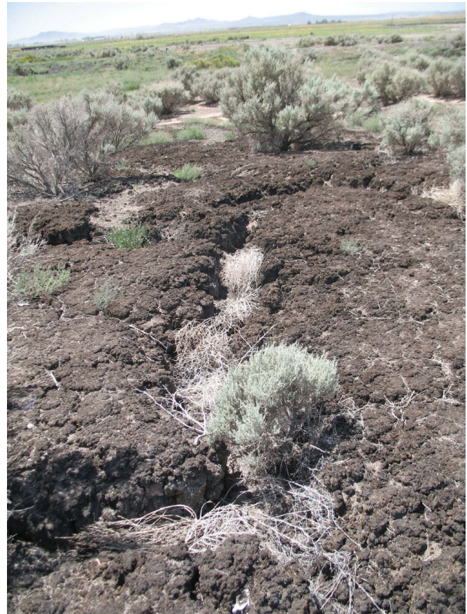
Figure 37. Vertical desiccation cracks developed in dried peat deposits on the east side of the Enoch graben in a former marsh area (view is to the northwest). Photo taken in June 2009.
