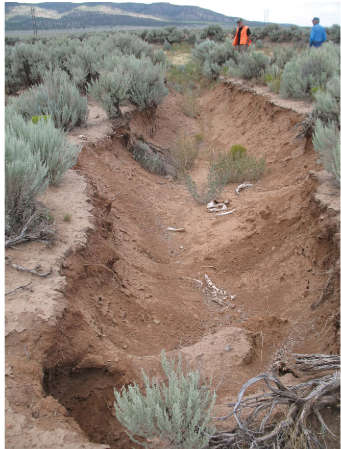
Figure 44. Gullied Quichapa-west fissure QWF4 where it crosses a stock pond (view is to the north). Photo taken in August 2009.
