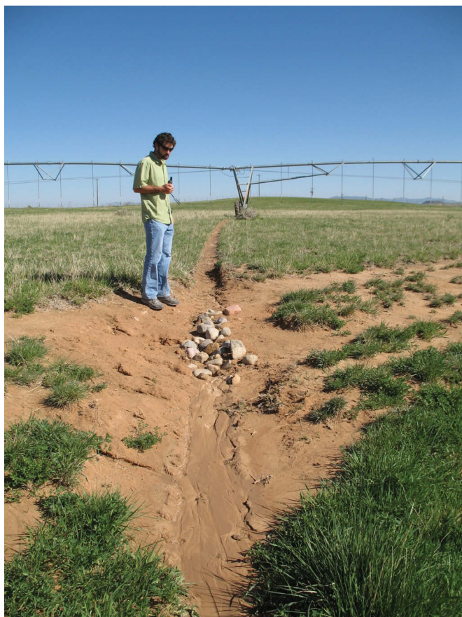
Figure 28. Repair to irrigation pivot track where it crosses the scarp of the EGWF1 fissure (view is to the northwest). Photo taken in May 2009.
