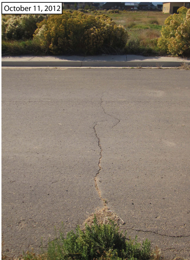
Figure 33 (above). Progression of crack formation on asphalt concrete pavement at 5200 North in the Legacy Estates subdivision in Enoch City. Cracks are coincident with the mapped EGWF3 fissure. View is to the south.
