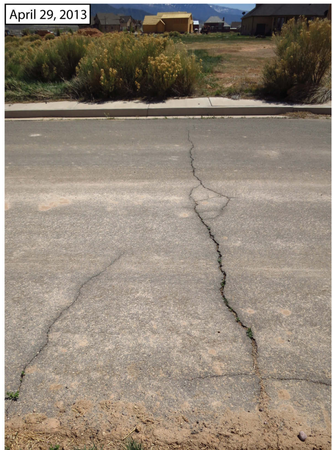
Figure 33 (above). Progression of crack formation on asphalt concrete pavement at 5200 North in the Legacy Estates subdivision in Enoch City. Cracks are coincident with the mapped EGWF3 fissure. View is to the south.
